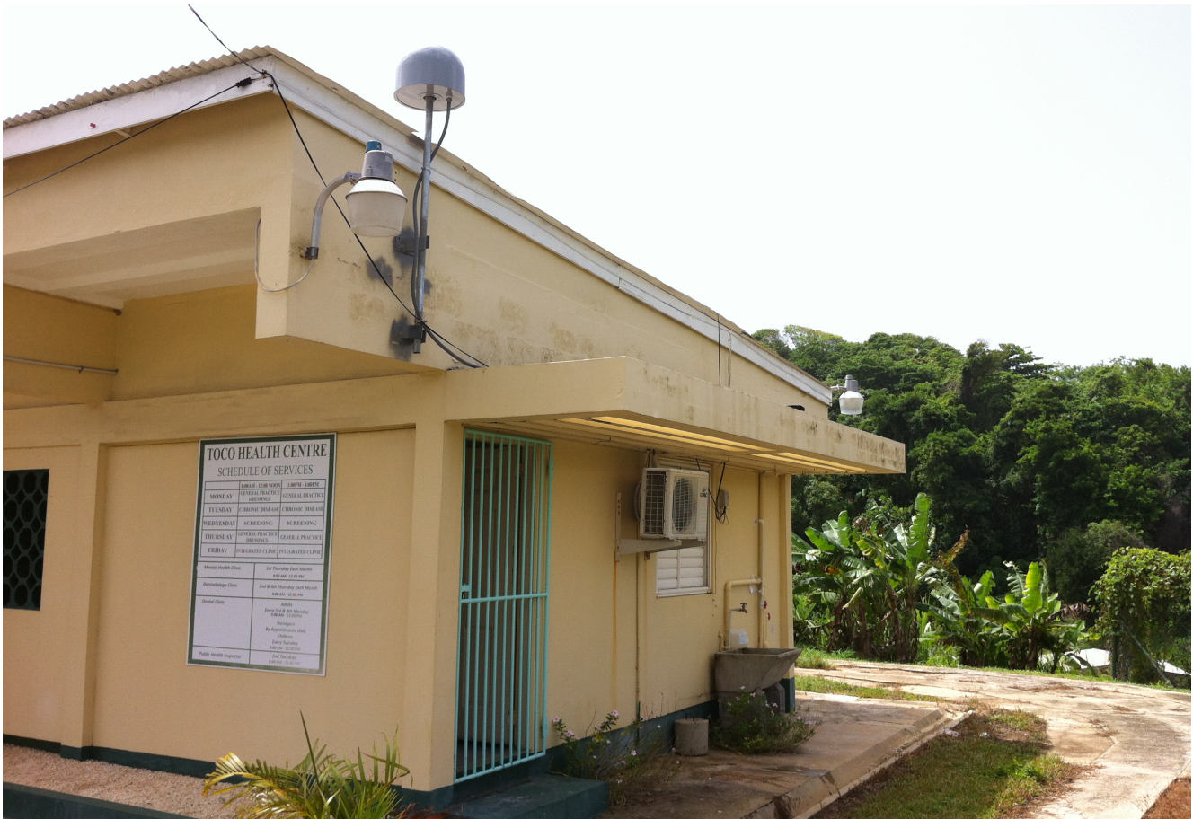
Figure 2. GPS monument located at the Health Center building in Toco, Trinidad.
