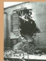
Burbank Elementary School
