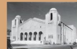
Reinforced masonry auditorium sustained little damage
