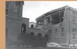
Five students killed when unreinforced masonry gymnasium collapsed
